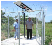
Effective theft protection: Panel and tracker fenced in and protected by barbed wire
